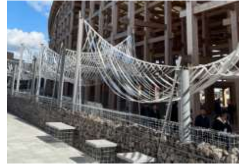
Sunshade built using scrap material from “SPACECOOL”
