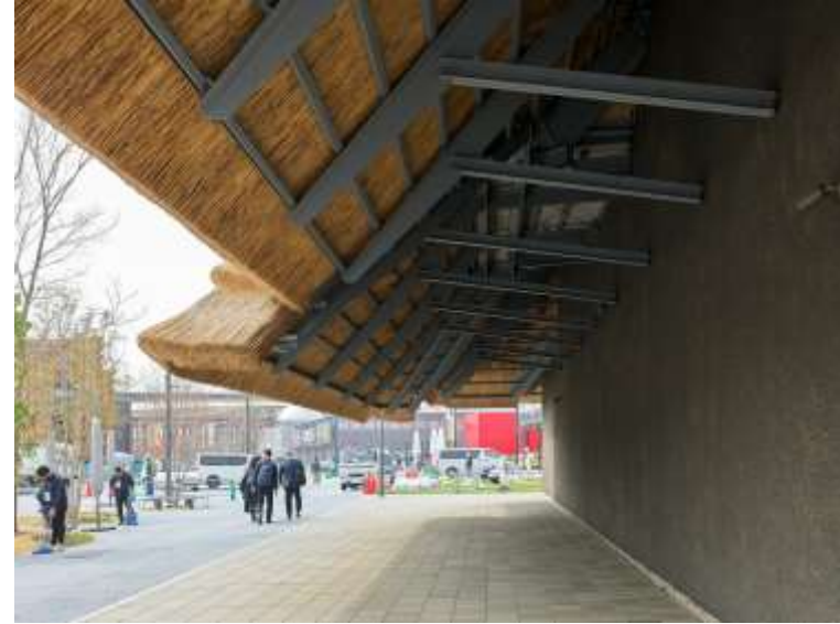
Wide space under the eaves One of the advantage of Steel structure
