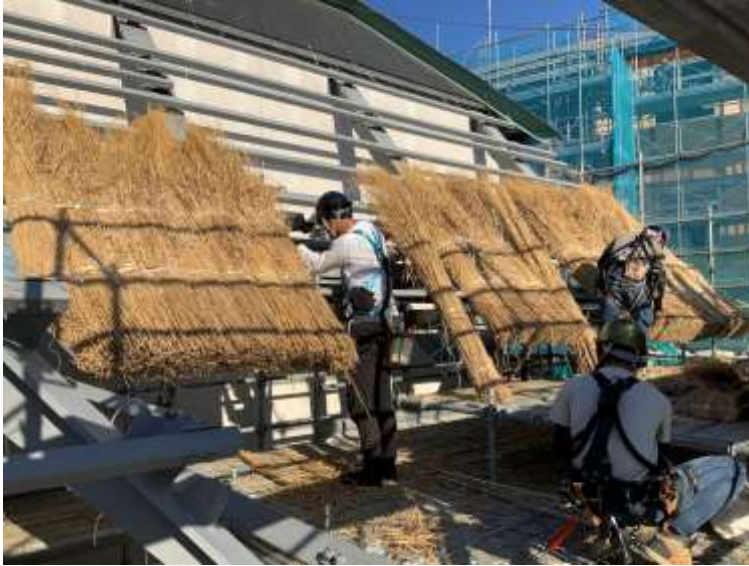
Installing thatched roof to the Steel frame base
