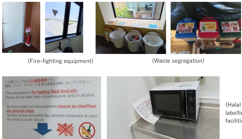
Figure 2-4 SUS Patrol On-site Inspection
