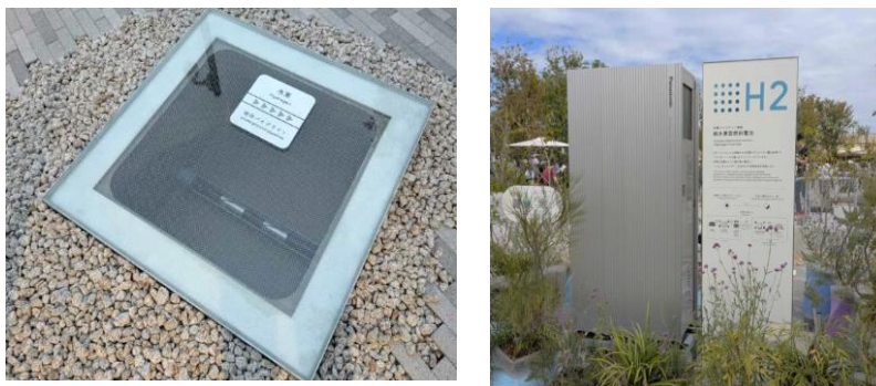
Figure 3-2-7 Hydrogen supply pipeline and the hydrogen fuel cells it supplies
